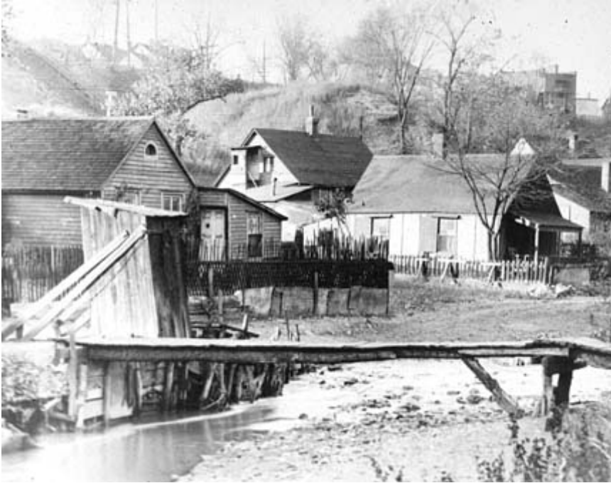
Illustration 9: There were no city services in the Hollow, so outhouses were hung over the creek to provide some sort of plumbing. The houses show many signs of modifications made by "jack-knife carpenters" who were famous for building "by guess and by golly." The cantilevered outhouses must have given big Swedes some anxious moments!
