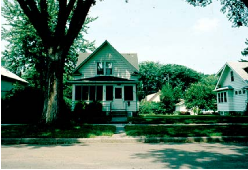
Illustration 13: This story and a half was built by a railroad machinist for his wife and three children. To save money the basement was added later.
